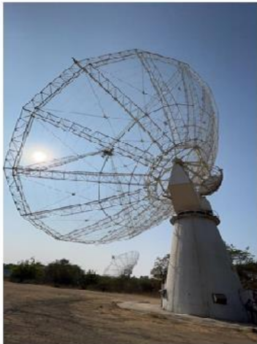
Parabolic dish with an outer diameter of 45m
